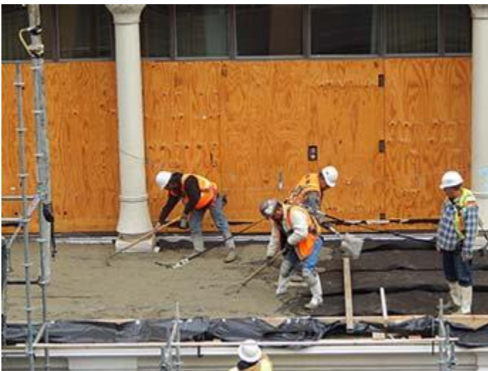
Workers with Chamberlin finish concrete on a Driskill balcony
